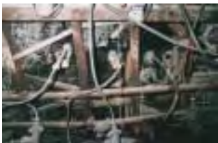
Gas drainage hole
